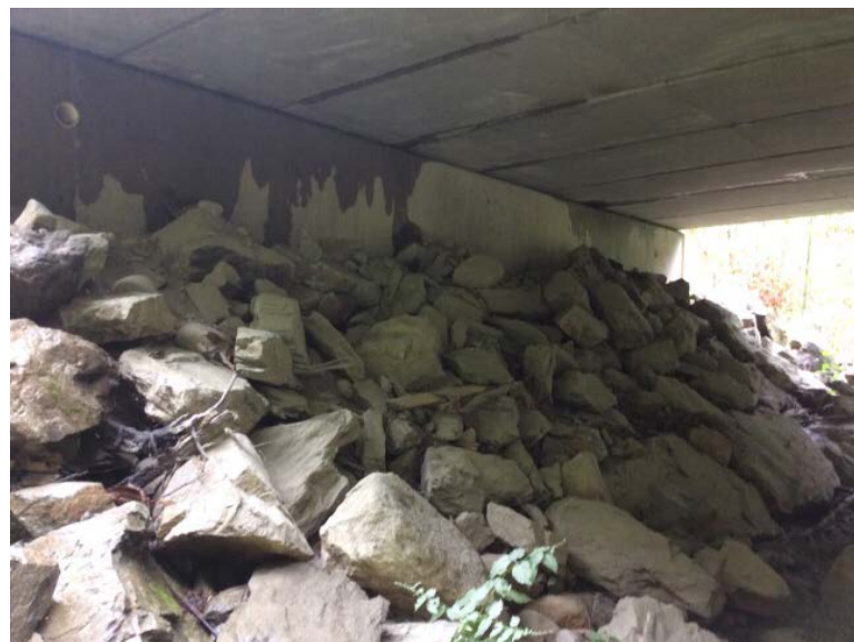
Left Bank Abutment when facing downstream
