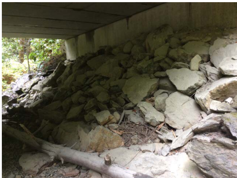
Right Bank Abutment when facing downstream
